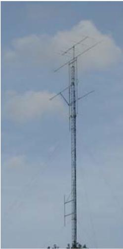
Stan's contest location is a hilltop in the Allegheny Mountain range at 2400 ft ASL. The tower is 155 ft of Rohn 55. It is located in the extreme NE corner of FN01, a stone's throw from FN02, FN12, and FN11.
